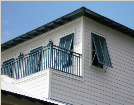
Figure 4-13. Bahama shutters made from durable extruded aluminum components add island flair to homes and provide effective opening protection. Source: Roll-a-way/QMI.
