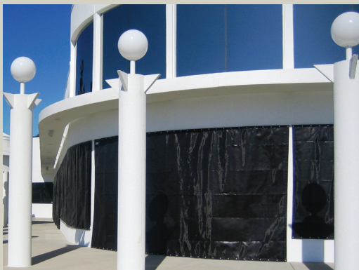
Figure 4-18. Polyethylene basket weave fabric windscreen deployed directly over ground floor windows of coastal home. Source: Roll-a-way/QMI.
