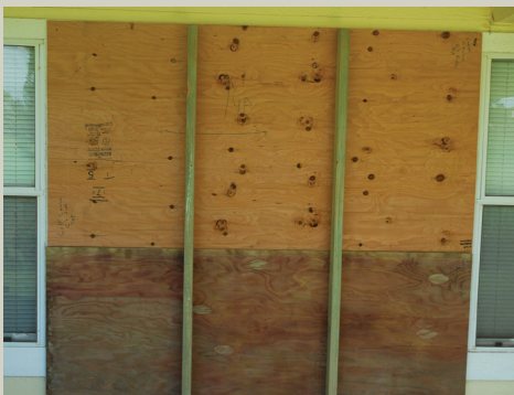
Figures 4-21 and 4-22. Not only is it necessary to install plywood opening covers correctly, it is also important to label them correctly and store them away from heat and humidity.
