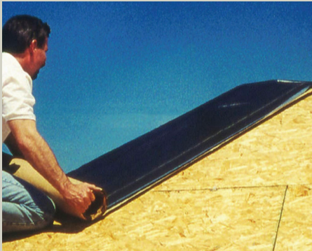
Figure 4-9. Synthetic underlayments are typically made from polypropylene, polyester or fiberglass fabric that weighs less than felt paper, can be manufactured with anti-slip surfaces and can withstand exposure to the elements for six months. Source: Carlisle Coatings & Waterproofing.
